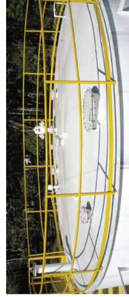
Figure 2.14: Fixed roof tank openings.
