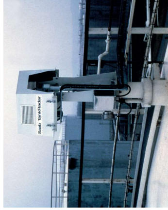
Figure 2.9: First high precision radar gauge installed in 1985 on a refinery tank.
