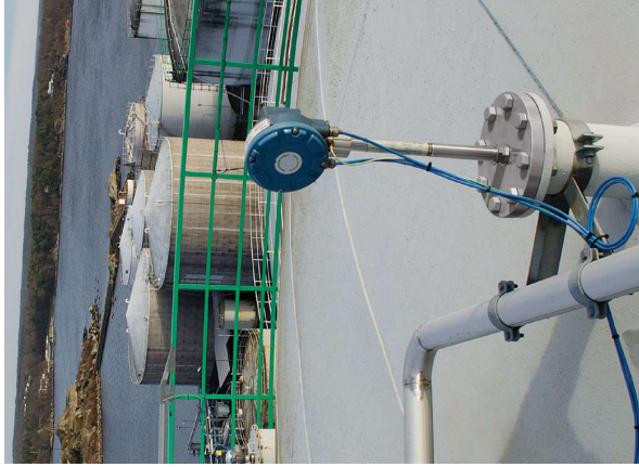
Figure 6.1: Top mounted temperature transmitter for up to 16 spot temperature elements.
